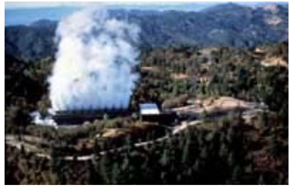
A geothermal heat utility in California.
